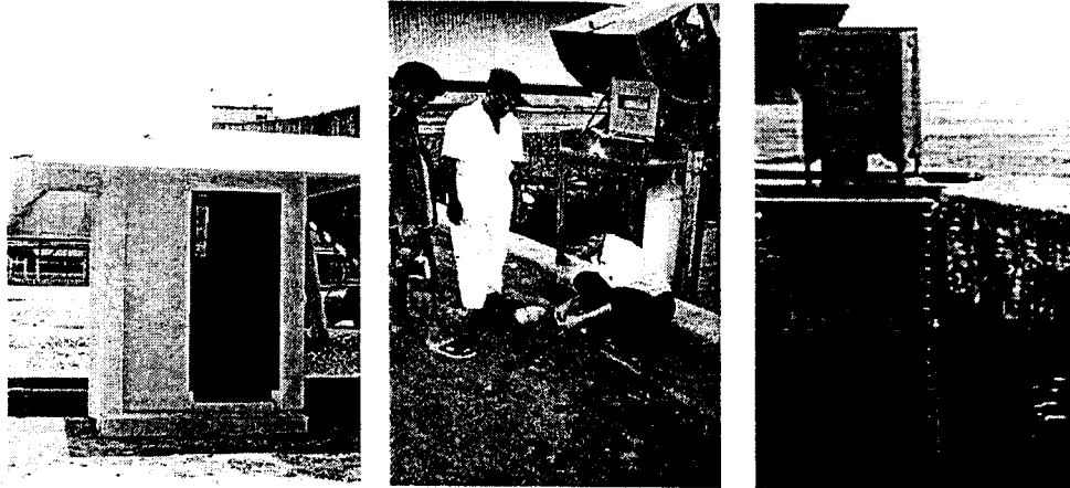
Figure 3. The existing tidal stations are still in different type of buildings. In the future the building should be standardized like the left hand building.
