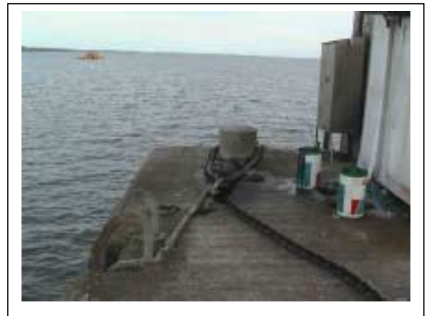
Plate 2.11 Gauge Control Box
