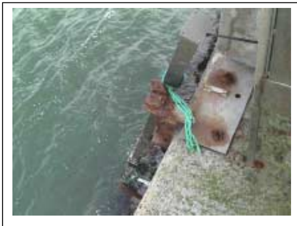
Plate 2.10 Conduit to Pressure Sensor
