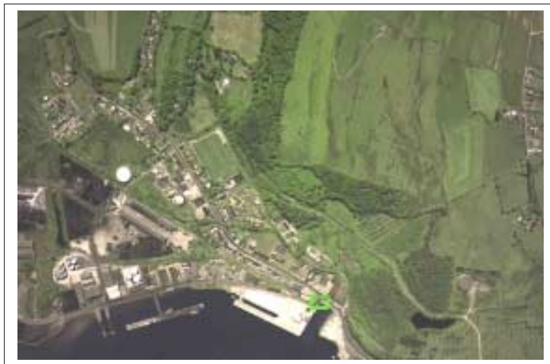
Plate 2.12 Foynes Jetty showing Gauge Location
