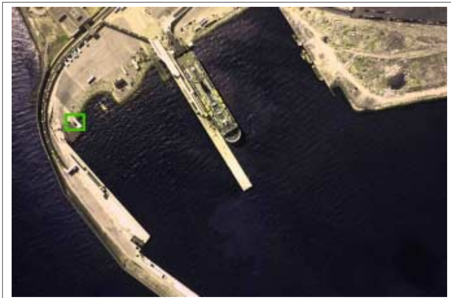
Plate 2.36 Rosslare Gauge Location
