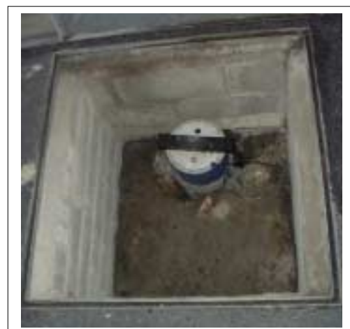
Plate 2.44 Acoustic Sensor
