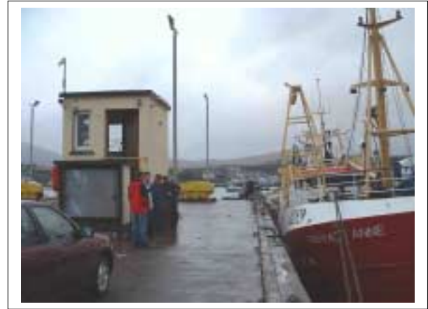
Plate 6.22 Syncolift Control Cabin
