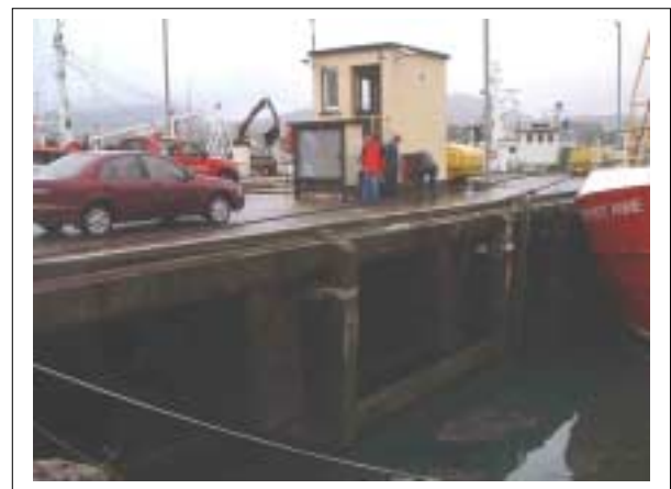
Plate 6.24 Jetty Structure and Control Cabin
