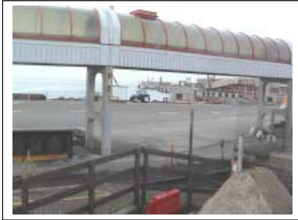
Plate 2.37 Rosslare Gauge Location (1)
