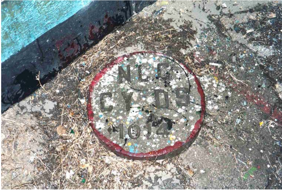
Figure 12 and 13. Bench Marks in Bushehr. The bench mark are located near the tide gauge and are tied into the Iranian levelling network
