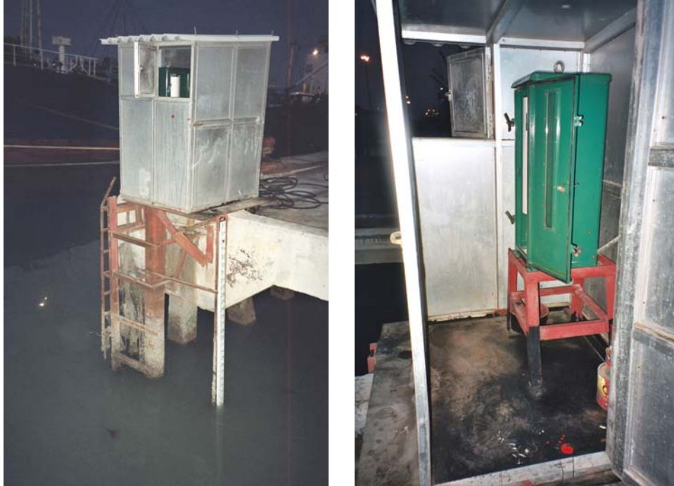
Figure 9 and 10. Float gauge (manufactured by the Ott company) in Bushehr.
