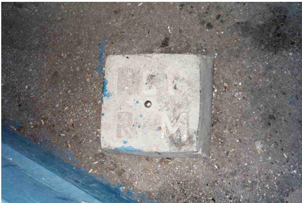
Figure 12 and 13. Bench Marks in Bushehr. The bench mark are located near the tide gauge and are tied into the Iranian levelling network
