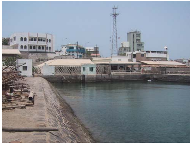
Fig 2. Port Control Tower, Tide Gauge hut (centre) and data logger hut (left of photo) with Pilots Pier on the right at Tawahi.
