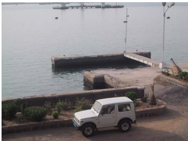
Fig 6. YPA Head Office Jetty (Jetty hand rails removed for repairs).
