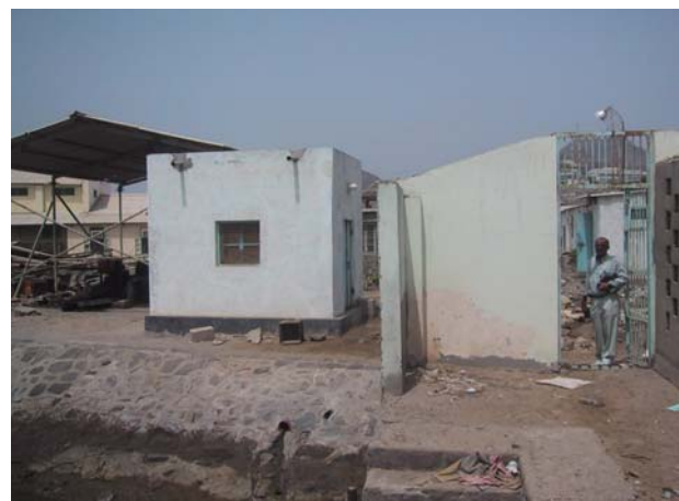
Fig 5. Adjacent watchmen's hut housing the WS Ocean-Systems data logger /printer/chart plotter, with Mahfood M Mohammed Kassim- Chief Hydrographic Surveyor
