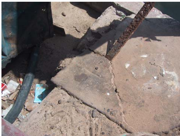
Figure 4. Tide Gauge benchmark-bolt in concrete surface with letters RA.
