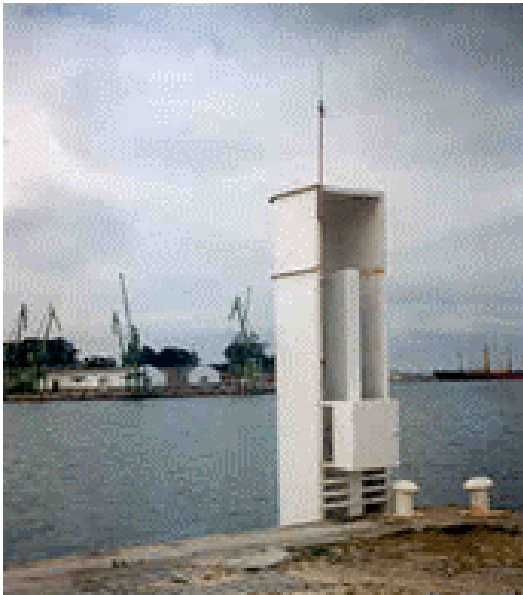
Figure 8 SRD station in the harbour of Vilagarcía de Arousa
